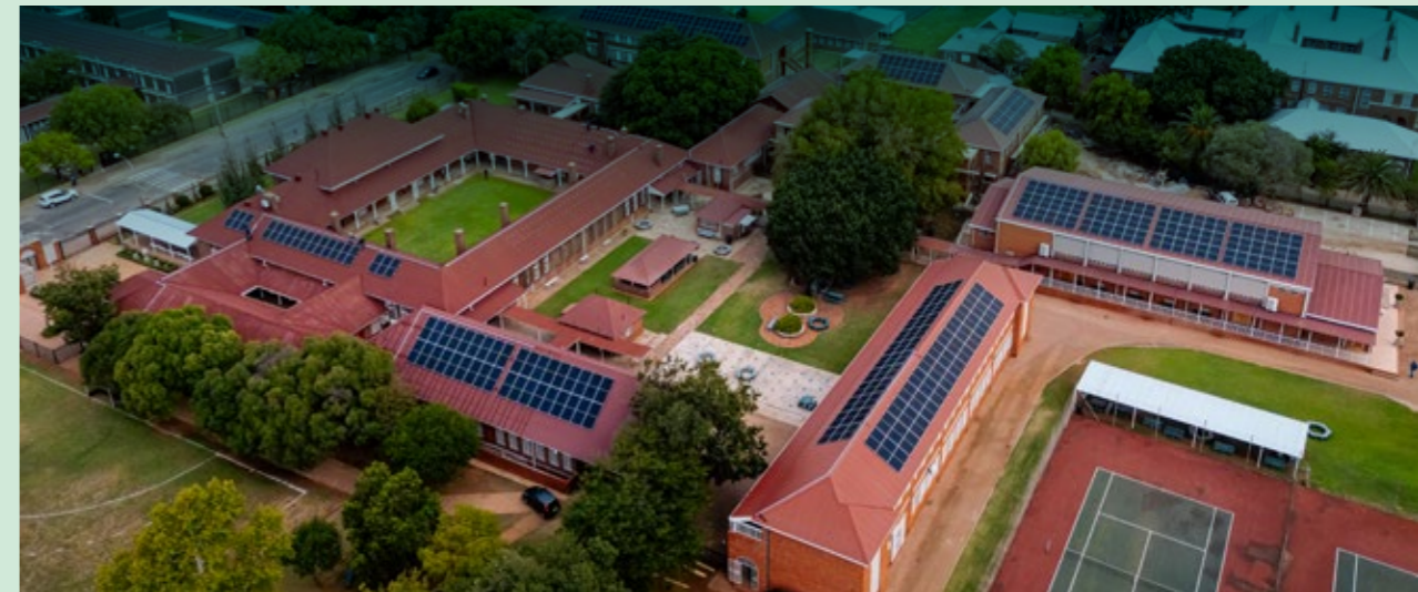
The High School for Girls Potchefstroom, 366 kWp, South Africa
